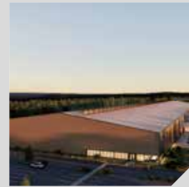
TIMBERLAB, USA 340,000 m 3 clean air per hour
