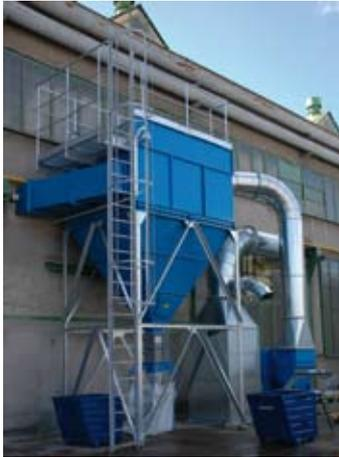
Cartridge filter for sand blasting unit
