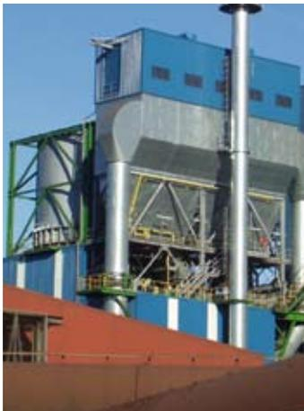
Pressure surge resistant filter for dedusting a coal grinding mill
