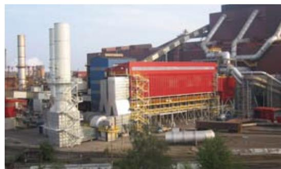
Chamber filter in the steel industry
