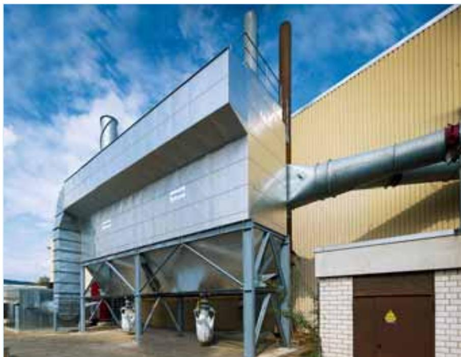
The exhaust air is collected using an enclosure for which Scheuch has determined the required exhaust airflow as a function of the bath surface and the customer's product mix. An energy-saving control program regulates the performance of the dedusting plant as a function of the production parameters.
