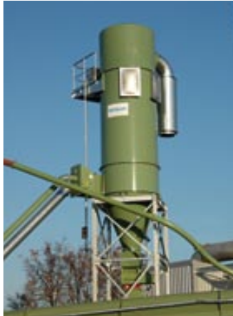
Circular filter in the wood processing industry
