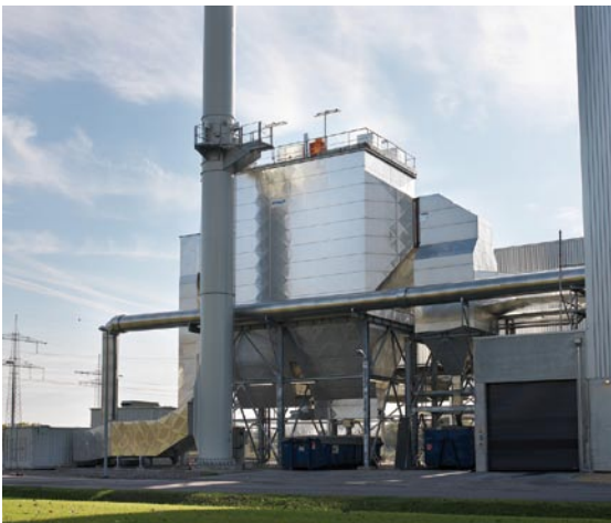
2-Field ESP with multi-cyclone
