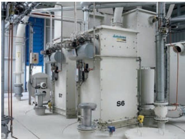
IMPULS Compact filter rated at 1,700 m 3 /h for silo air extraction.
