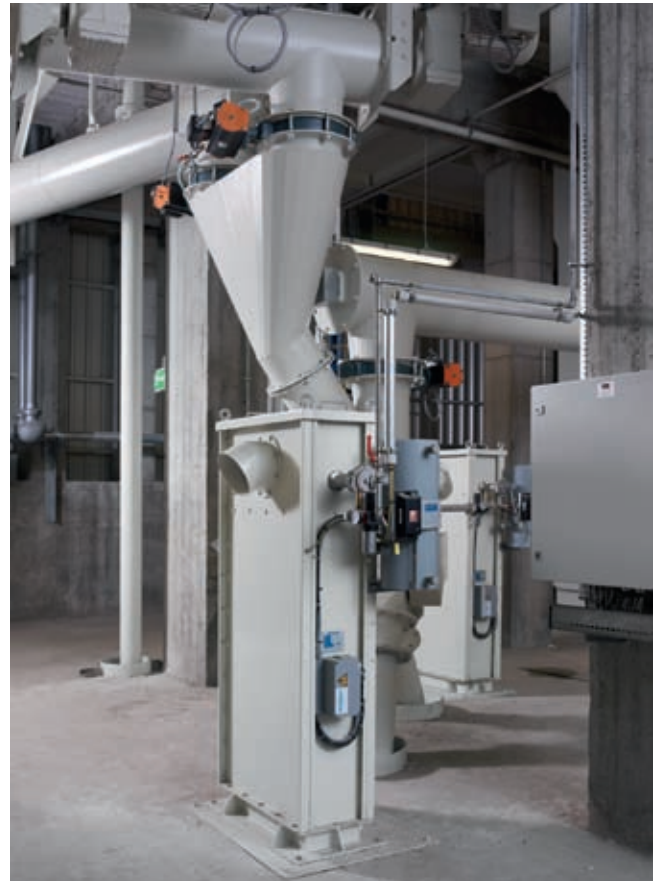
The IMPULS Compact filter program covers the performance range from 200 to 30,000 Am 3 /h.
