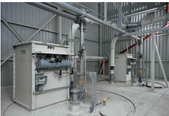
The IMPULS Compact filters are pre-assembled and delivered ready for connection.
